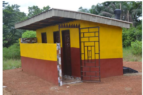
Mfuma: The finished toilet block containing three Enviro Loos
