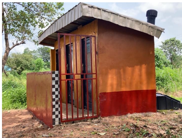
This block of Enviro Loo toilets now provides a clean and safe place to go to the toilet.
